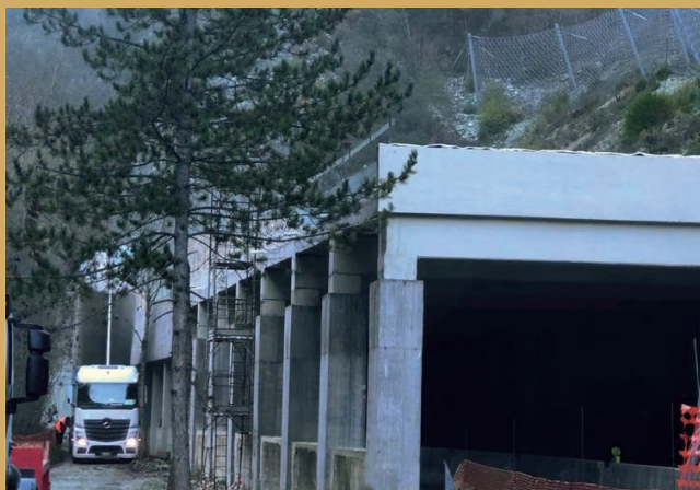
Norcia (PG) - Galleria paramassi
